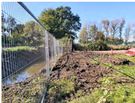
Above: Work on the Burntwood Gateway in progress [DG Chick]
